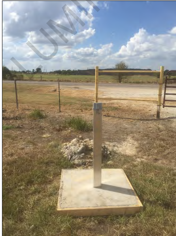
Photograph 2: BAP-58 prior to installation of bollards.
