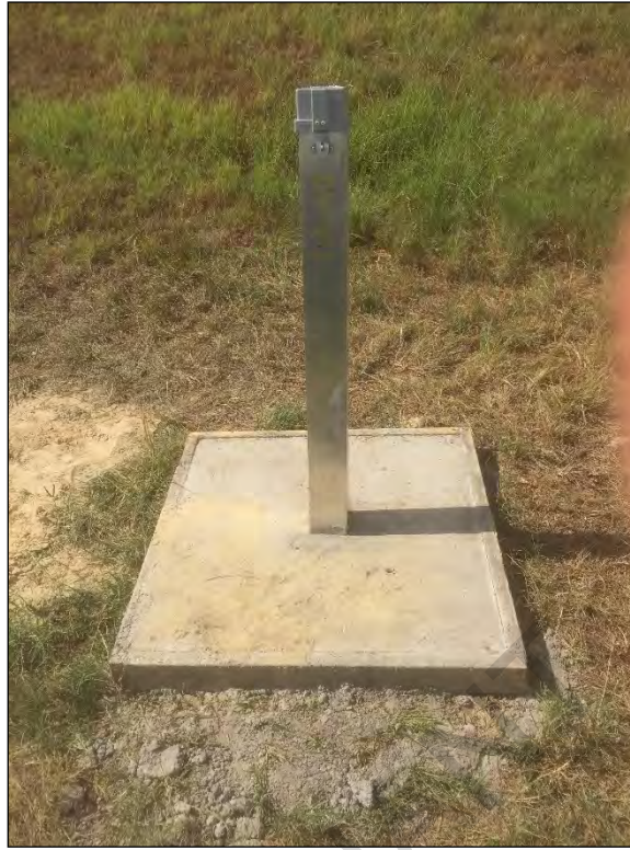
Photograph 5: BAP-61 prior to installation of bollards.
