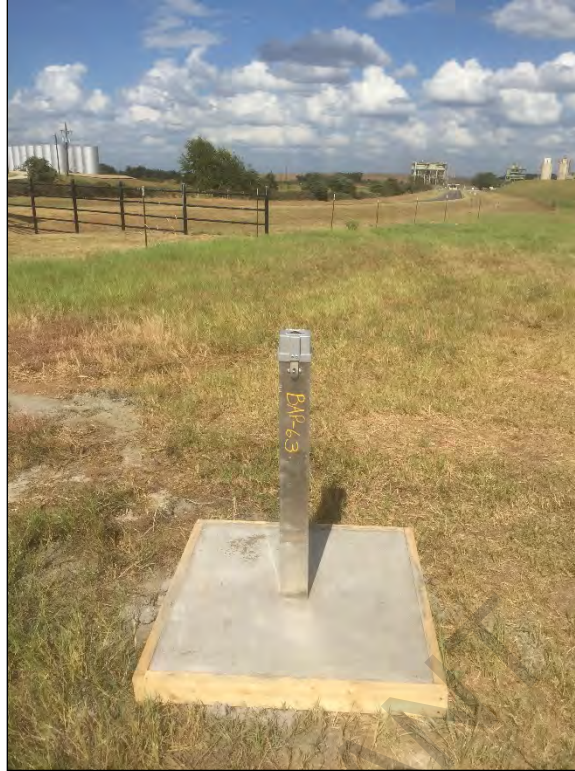
Photograph 7: BAP-63 prior to installation of bollards.
