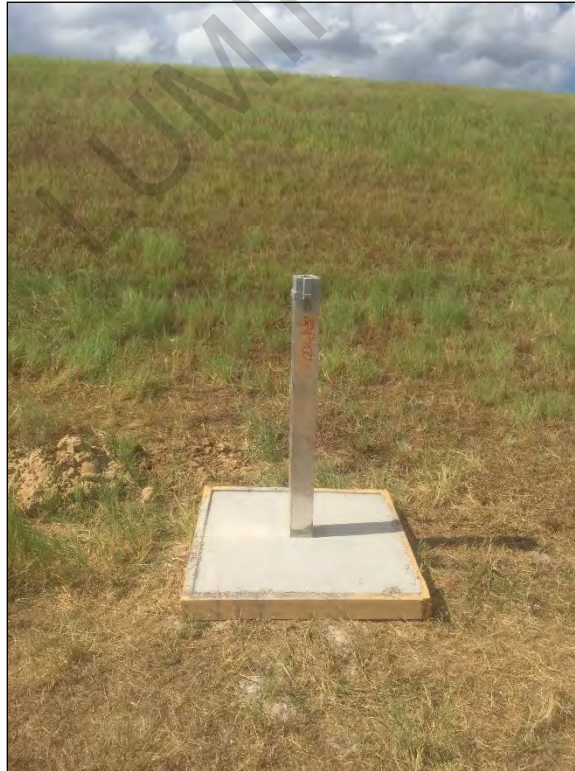
Photograph 4: BAP-60 prior to installation of bollards.
