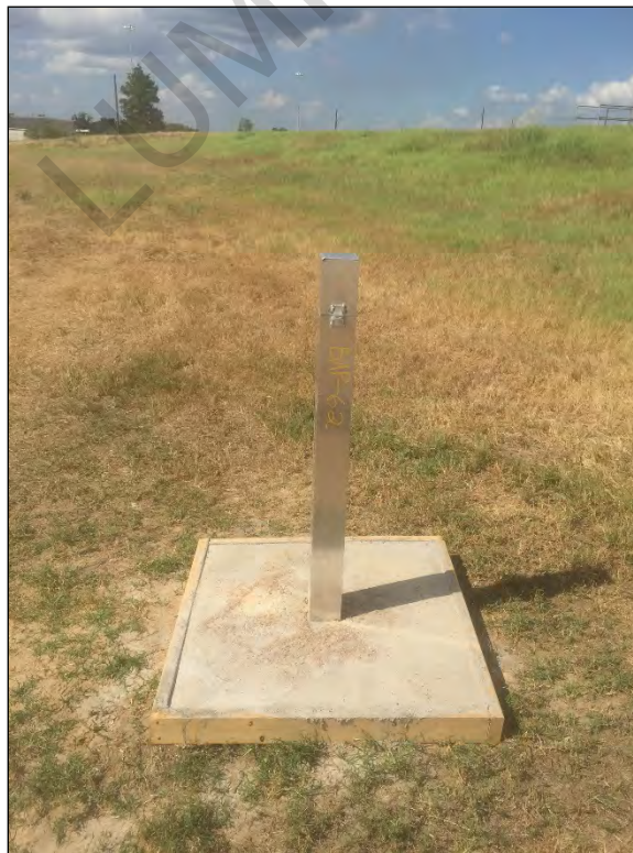
Photograph 6: BAP-62 prior to installation of bollards.
